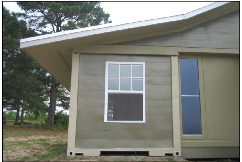
This Rural Studio house for families, developed by AIDS Alabama, Auburn University, and AIDS Outreach of East Alabama, uses railroad cars for bedrooms.
